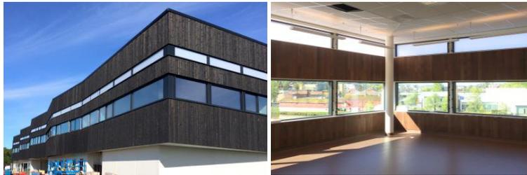
Fig. 6. Levanger primary school, Norway. The entire second floor has built with two glazing systems: aerogel glazings for upper windows and normal clear glass glazings for low windows [21].
