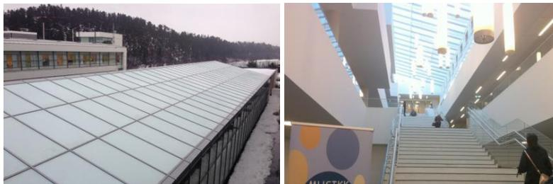
Fig. 7. Sandvika knowledge center, Oslo. The roof has been integrated with aerogel glazings [21].
