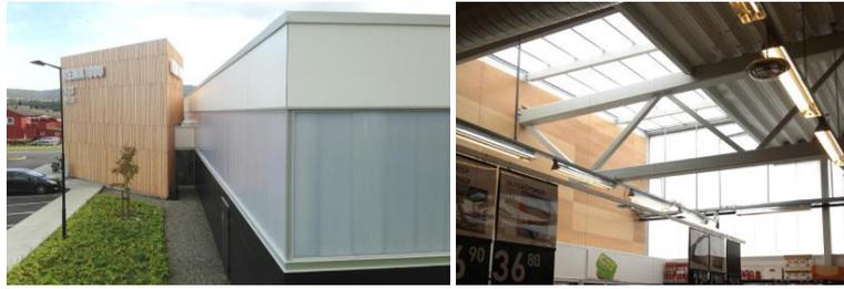
Fig. 5. The Rama 1000 supermarket at Kroppanmarka with 220 m<sup>2</sup> aerogel glazing panels [19, 21].
